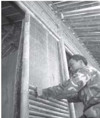
*Image 1: Building a wall with horizontal culms*
