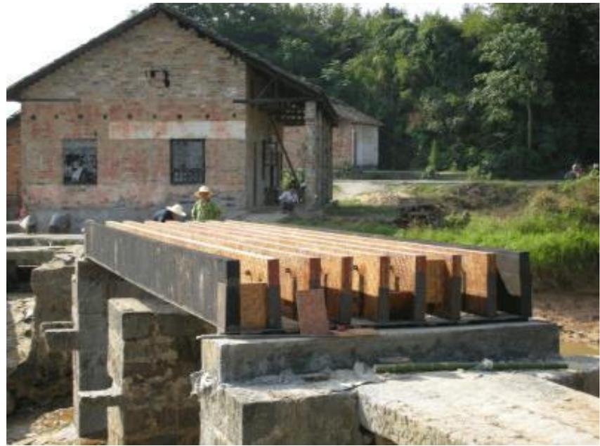
*Image 17: Bridge built using GluBam*
