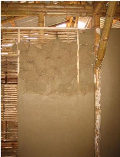
*Image 2: Wall made from plastered „esterilla”*
