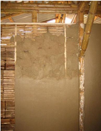
*Image 2: Wall made from plastered „esterilla”*
